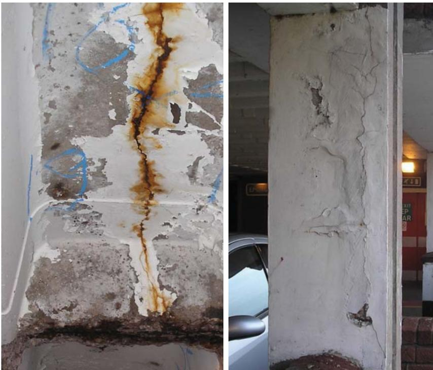
The effects of chlorides in concrete are exacerbated by advancing carbonation and low concrete cover, symptoms found on this MSCP in the Midlands by **Martech** testing staff. Following an extensive concrete condition survey, **Martech** submitted a detailed report together with repair solutions.
