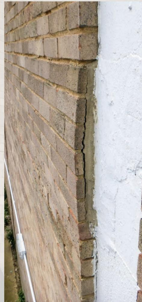
Martech was requested by a long-term client to assist with survey works on a large industrial building. Specifically, this involved a south-facing brick-faced wall with bulging and various other signs of distress.
