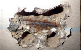
The original concrete condition survey brought to light some issues in the design and construction of this structure in south-east England, dating back a number of years. Amongst the findings was the presence of HAC concrete in parts of the construction. Martech involved a Structural Engineering practice familiar with such structures for further phases of works and analyses, which are ongoing today.
