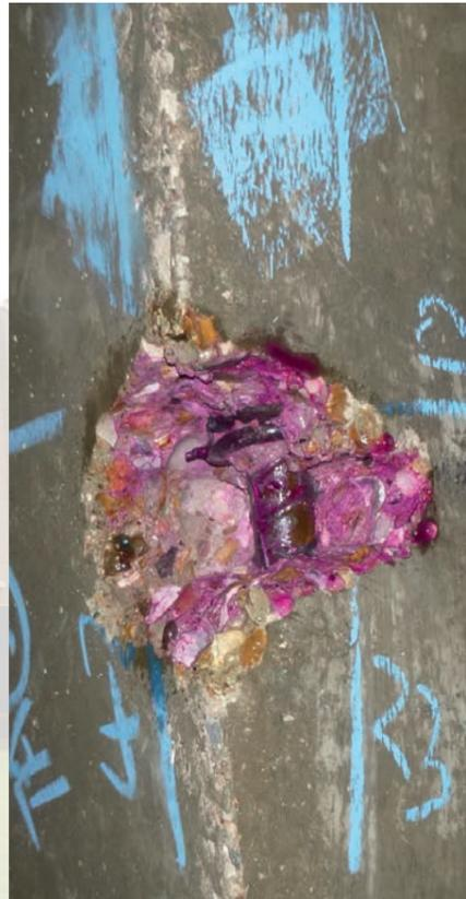
There were classic signs of concrete distress as a result of reinforcement corrosion and a detailed appraisal of all typical elements of all the structures was needed in order to understand the relationship between concrete cover, carbonation and chlorides. Martech also took cores for petrographic analyses and compressive strength testing to build up a complete picture on concrete condition. Incidental numbers of samples were additionally
